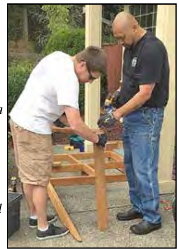
Left: 751 Volunteers on the finished Puyallup ramp built for the brother of a member.
